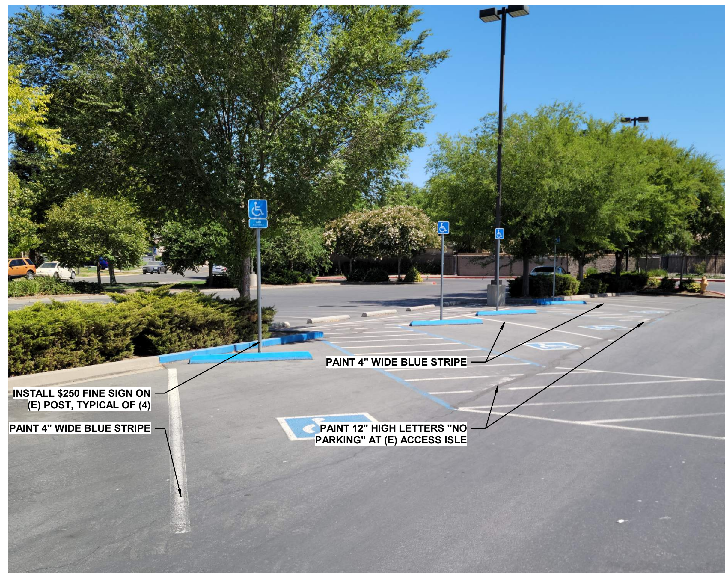
EXISTING ACCESSIBLE PARKING 12" = 1'-0" 2
